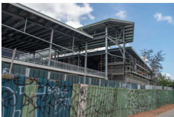
Gordons market under construction (2018)
