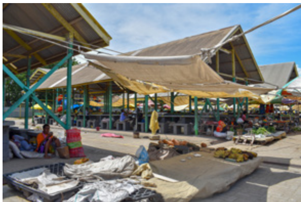
Gerehu market infrastructure (2018)
